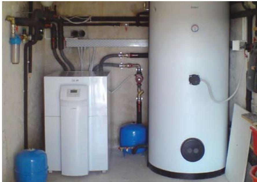
Sustav grijanja i pripreme tople vode geoTHERM VWS 460/2 s multispremnikom spremnikom alISTOR VPA 1000 u Molvicama
